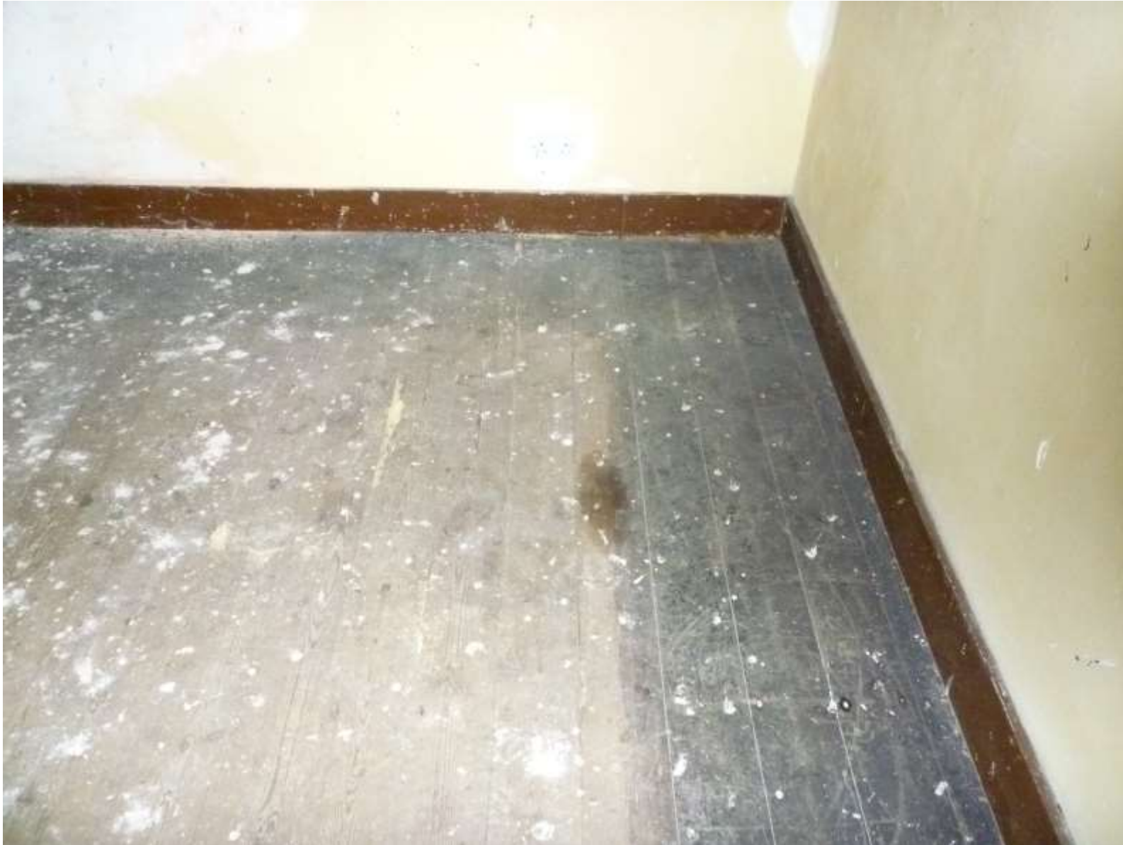
116. Bedroom 4 Floor in NE corner above blocked off stair case outside waiting room (see pic 18). No sign of access 'patch' indicating whole floor must have been replaced since stair access was blocked off.
