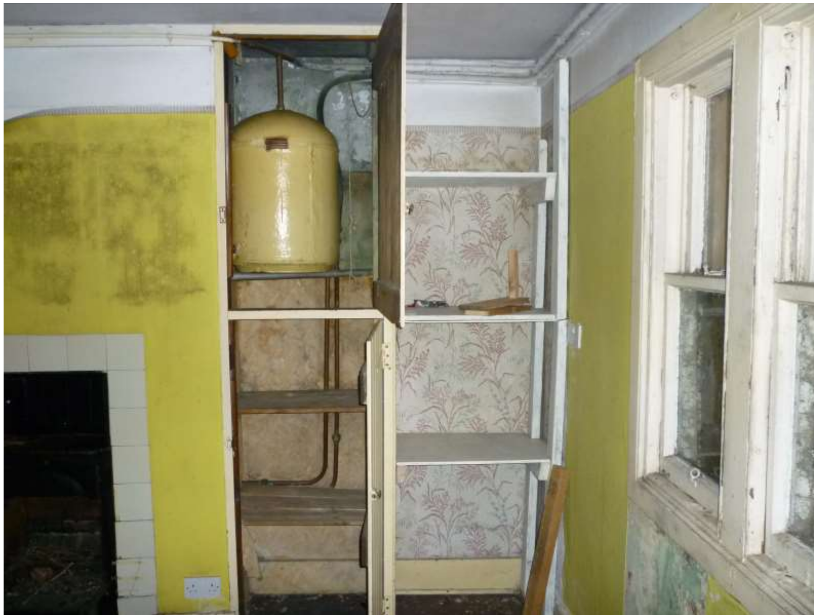
68. Alcove to right of chimney breast showing cupboards and hot water cylinder heated by adjacent kitchen stove
