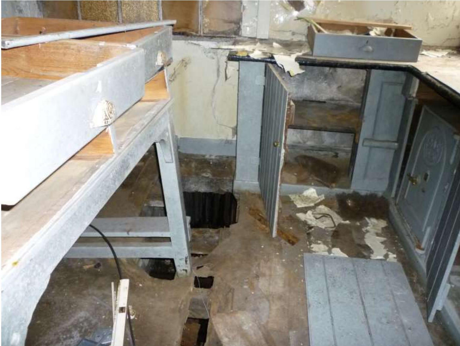
55. Rotten floor reveals hole under west wall. There was once a point or signal lever in the office with under platform tunnel for trackside connection
