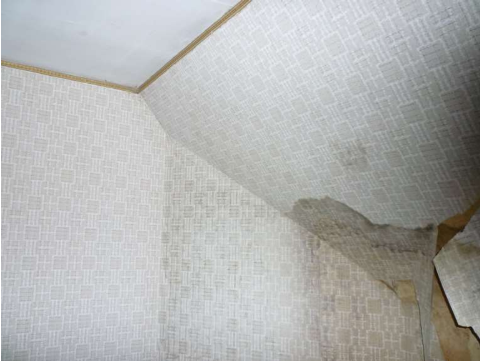
99. Bedroom 1: angles of walls and ceiling above fireplace (as well as long term roof leak)
