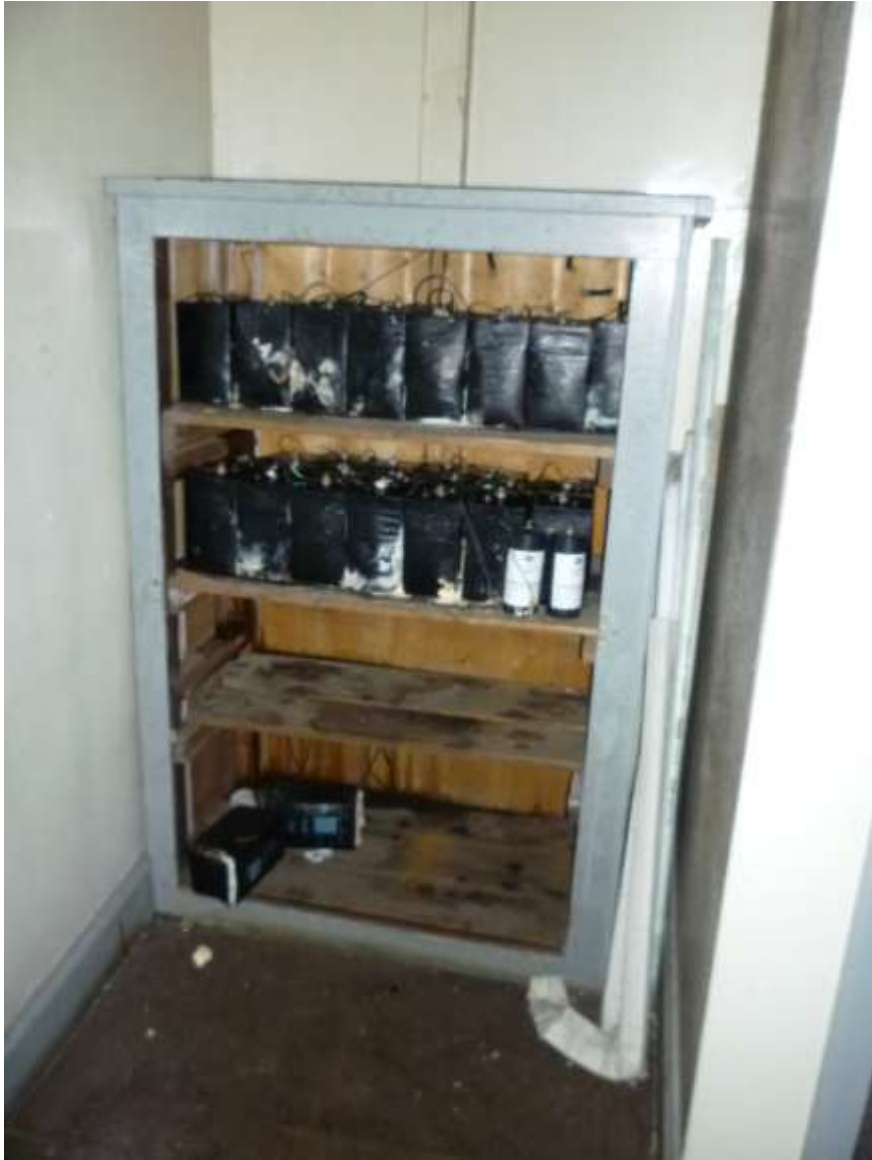
42. Cupboard of corroding British Rail batteries against the south wall (#8). It is believed that there was a door behind leading from the store (stationmaster's office) to the entrance hall or the stationmaster's house
