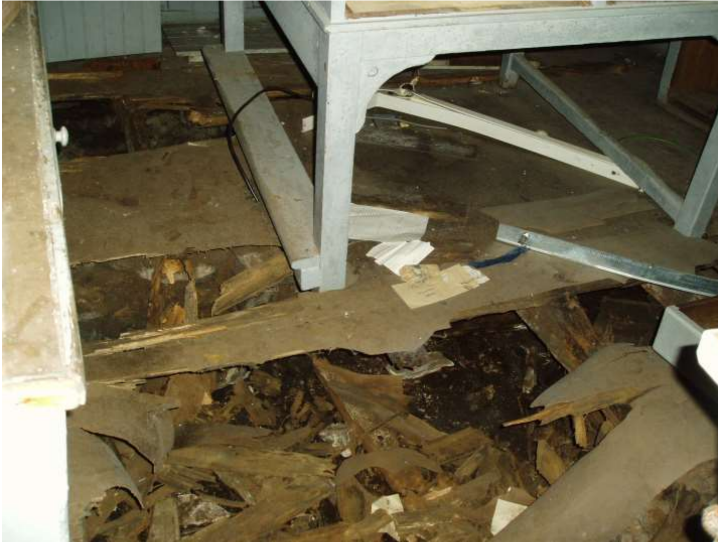
35. In both the office and the store, the suspended floors are rotten and very hazardous. This has restricted the photos in these two areas.
