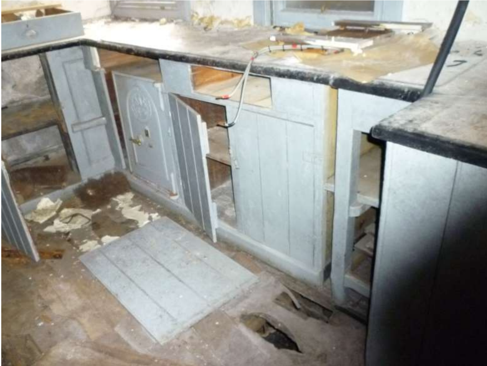
48. Counter, cupboards, safe and rotten floor below north windows in office
