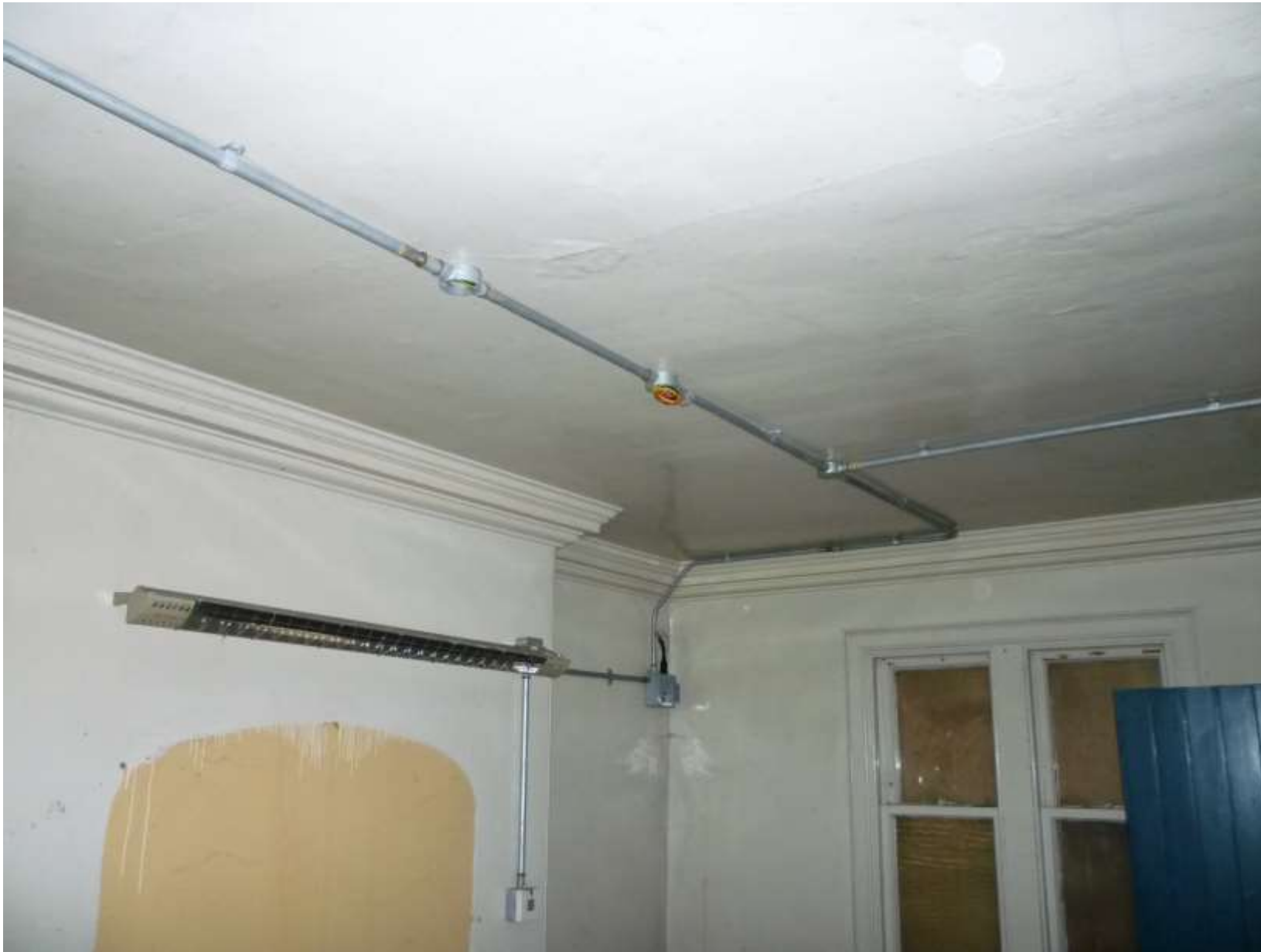
27. Waiting room ceiling showing ducted electric cables and outline of lost over mantle / mirror
