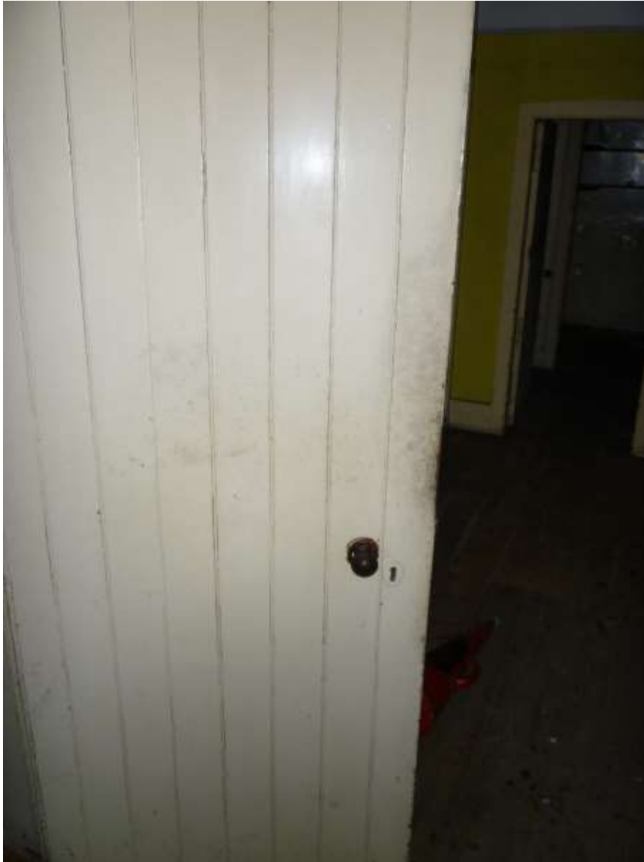
71. Door into hall from kitchen – hall side. All internal doors are of this type except bathroom door with glazed panels and door between bedrooms 3 & 4
