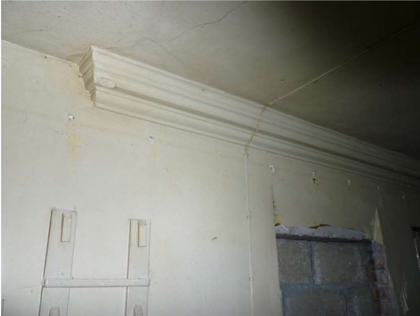
43. Cornice in store (Stationmaster's office, west wall); the only room in the building with a decorative cornice apart from the (first class waiting) room. See pic 26
