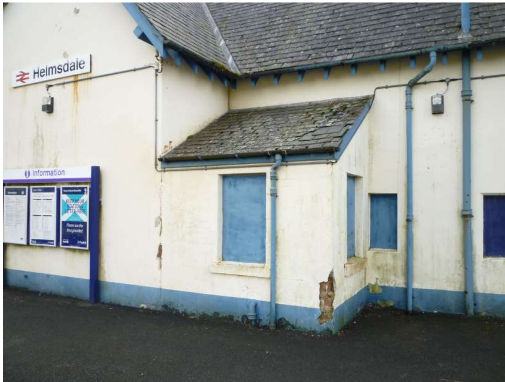
12. East elevation showing detail of scullery annexe, added at unknown date. Behind the damaged render it can be seen that this is brick built, unlike the concrete construction of the rest of the building.
