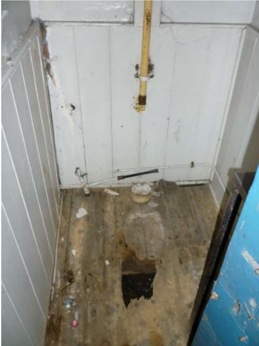
30. Looking in to off-waiting room toilet (rotten floor prevents access, but note aluminium wash basin behind door)
