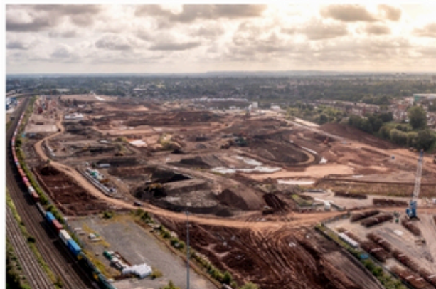
The HS2 Washwood Heath Depot under construction in Birmingham
