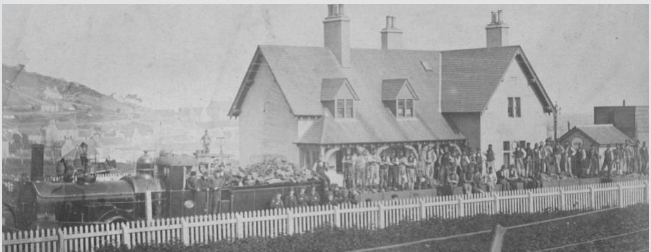
Dating evidence from the locomotive: Identified as No 40 (Keith), a Medium Goods locomotive built in 1864 and here in its original form. Rebuilt in 1885. The number of men standing on the wagons suggests these were construction navvies and not just a maintenance gang.
