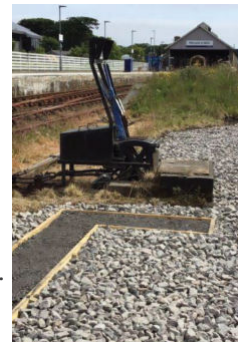
[Right] Safe access provided to a groundframe used for controlling points in the yard.
