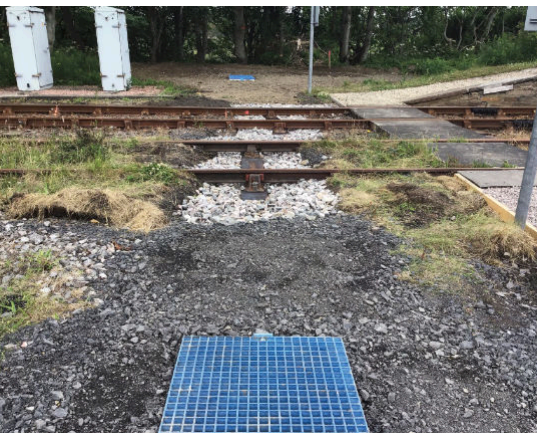
[Left] Reinforced UTX (Under Track Crossing) drainage pipes pass beneath the track. The blue cover is for access to a catchpit, used to collect silt and debris in a sump. Fifteen new catchpits were installed.
