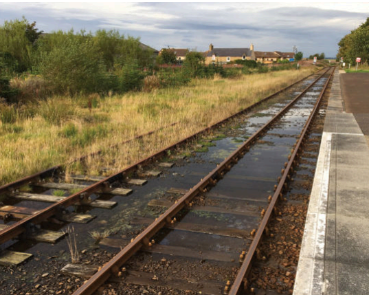
[Left and Above] The area before work commenced, the lying contaminated water revealing the extent of the problem.
