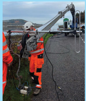
Attaching the aerial to the crane
