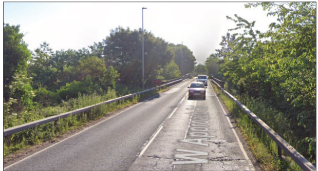
A part of the West Approach Road, Edinburgh - a former double-track section of railway. Barely room for a single carriageway road - this shows why it wouldn't have been simple to convert the single-track Far North Line.
