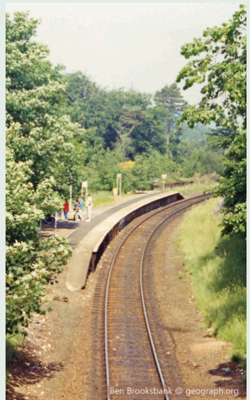
Culrain Station, from where the Lochinver line would branch off the FNL (1986)
