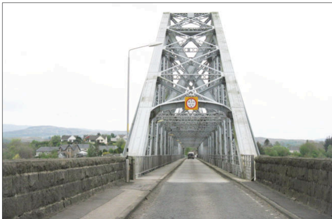
Not the most desirable use for a railway bridge!
