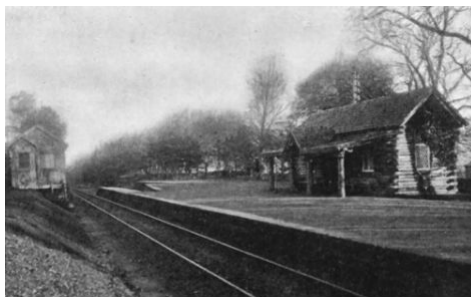
The original station building at Dunrobin
