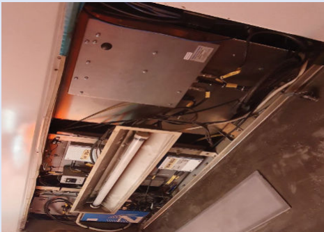
Equipment installation area in carriage roof
